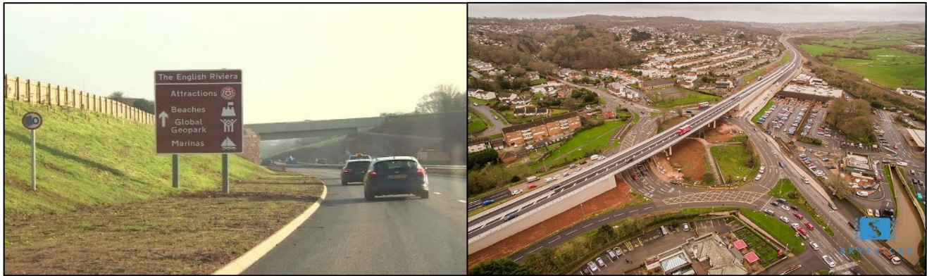
Figure 8: South Devon Link Road including flyover of Penn Inn roundabout
